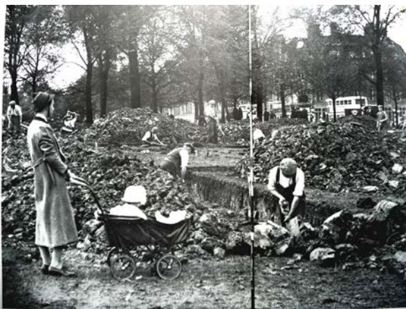
Trenches being dug on Streatham Common in September 1938 in preparation for protection from bomb blast. From London in the Twenties and Thirties From Old Photographs, by James Howgo, Batsford 1978.
