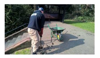
again. We edged the lawns back to their original line, removing old turf. This revealed soak away drains which had been covered by turf for years. Nick has spent days clearing the clogged-up silt in these
