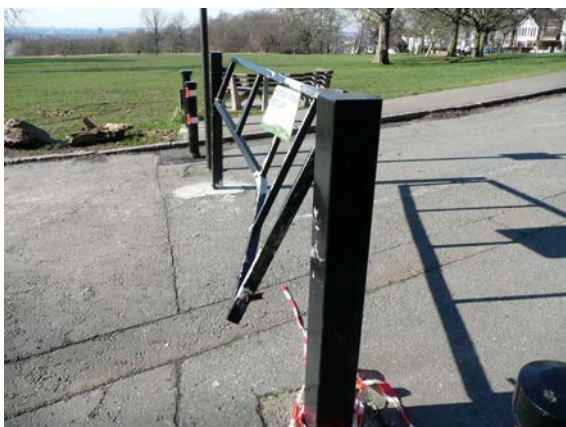
Drivers frustrated by this barrier sometimes remove the tree trunks positioned along the Common's edge and drive over the grass. A dim driver, in a stolen car, tried to ram the barrier - still not repaired - over the Christmas holidays.
